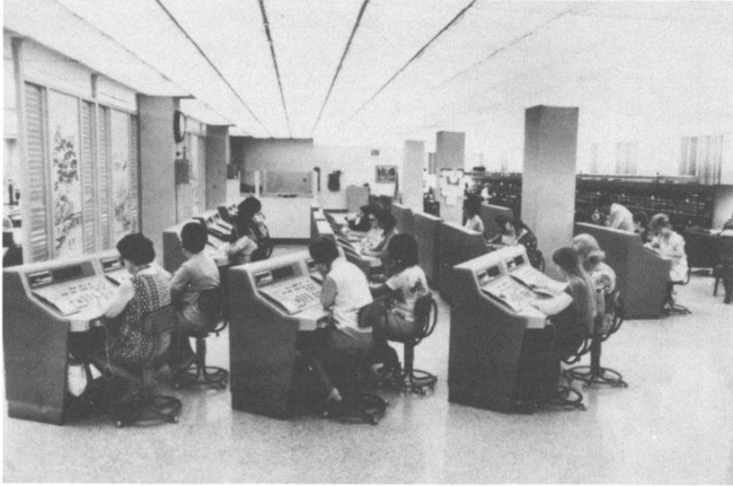
Fig. 1.—The old and the new: Traffic Service Position Systems replaced cord switchboards (far right) in Morristown, New Jersey, 1969. (Courtesy AT&T Archives.)
